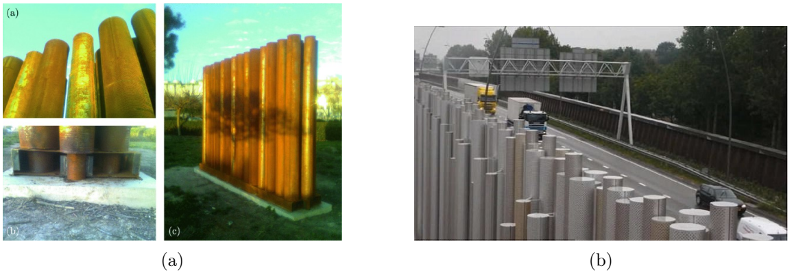
Figure 1.6: Examples of sonic crystals applications related to biomedicine and human health protection: a) Sonic crystal acoustic barrier (from [12]). b) Periodic pipe noise barrier installed in Eindhoven by Van Campen. (from [24])
