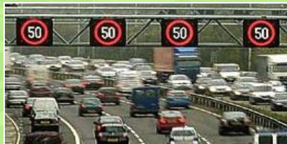
Example of a VSL installation on highway
